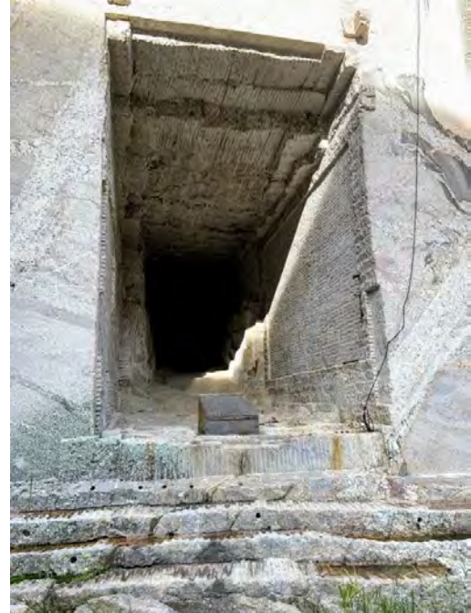
Photo 4 The actual Hall or Records was used by the crew to operate the firing control panel. Note there is no Means of Egress, Exit or Means of Escape. [Photo credit: NPS]
