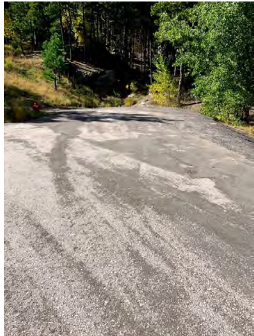
Photo 31 The Amphitheater Road Discharge Site likely will need to remain open and available for emergency access and fire equipment providing fire protection to MORU
