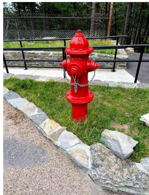
Photo 45 MORU has water access and capabilities, but it is limited to around the buildings at the base of the mountain.
