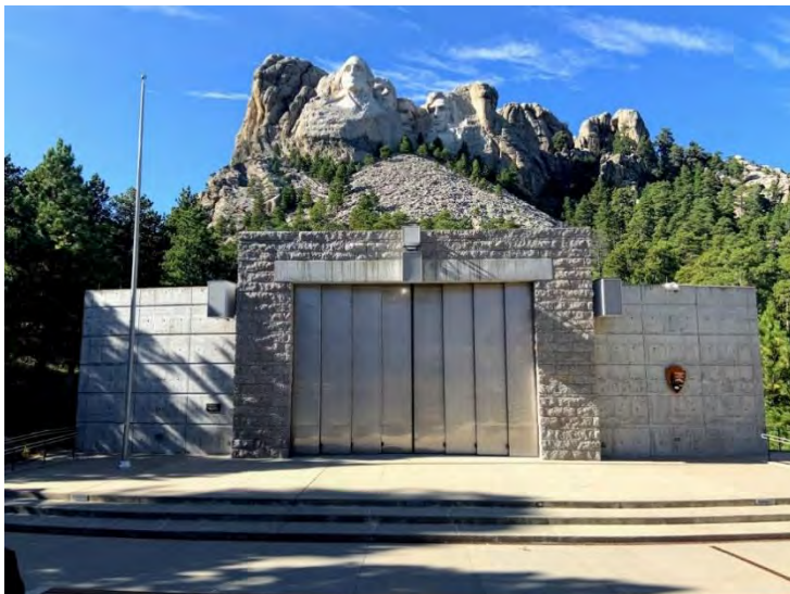
Photo 27 The Amphitheater stage and backstage with the MORU carvings above could serve as a discharge site for some articles pyrotechnic. Any proximate pyrotechnics here would need to be designed around whatever other programs and entertainment are conducted here on the day of the Show. Note: The view of the carvings from venter of the first three rows is blocked by the backstage. Other locations have the view blocked by tree branches.
