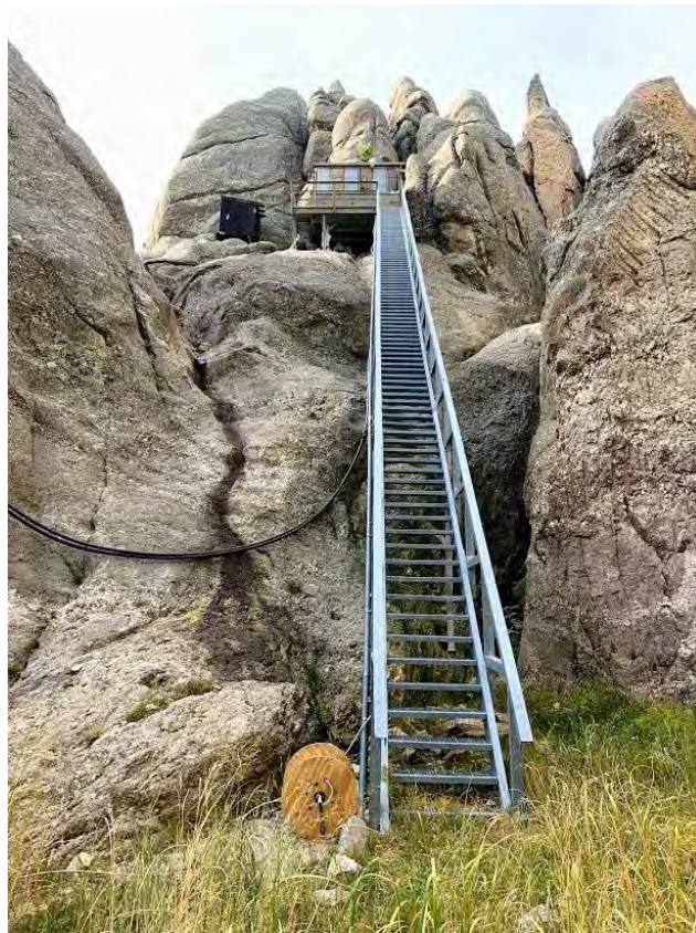
Photo 48 The metal steps up from the Hall of Records Canyon to the Guard Shack. Articles pyrotechnic holders could be secured to the outside of this structure.
